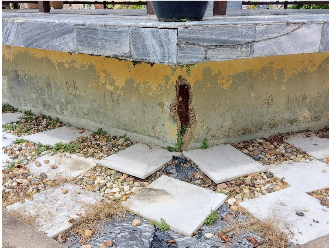
Cracked base of Mother Mary's Shrine
